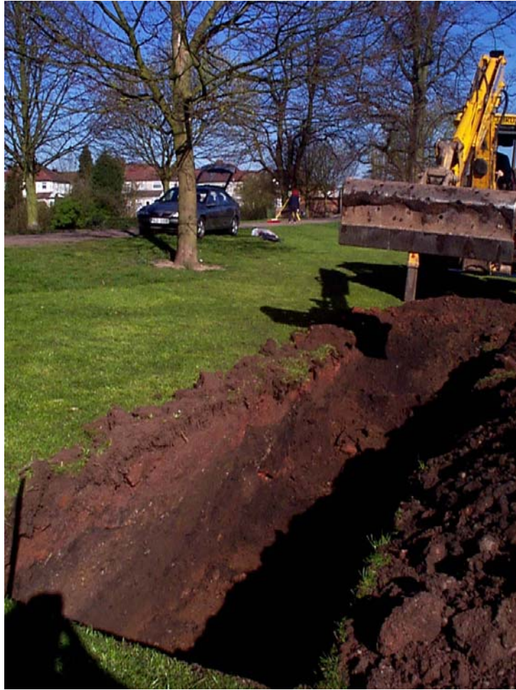
Fig. 4: Machining of Trench 1
